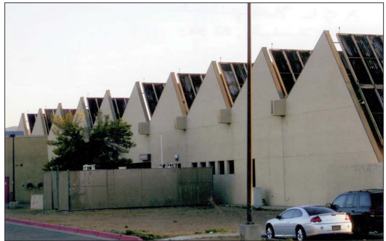
The ACL Hospital in San Fidel, New Mexico
